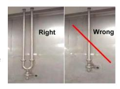
All dead ends must be eliminated. When a dead end is found, it should be cut out and replaced with straight pipe.
